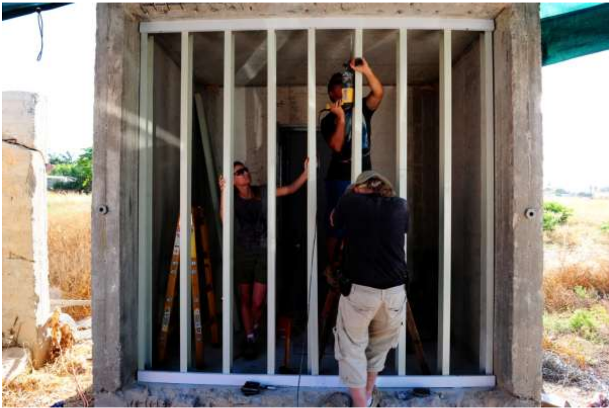
Figure 23 Glass fibre reinforced plastic wall target under construction
