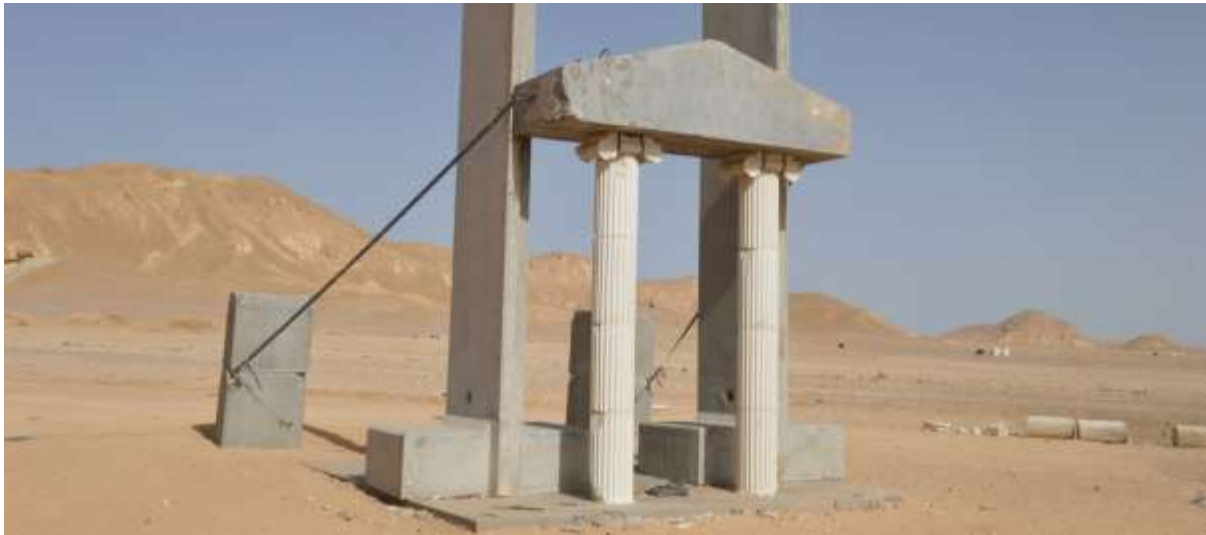
Figure 42 Neoclassical multi-drum columns after test
