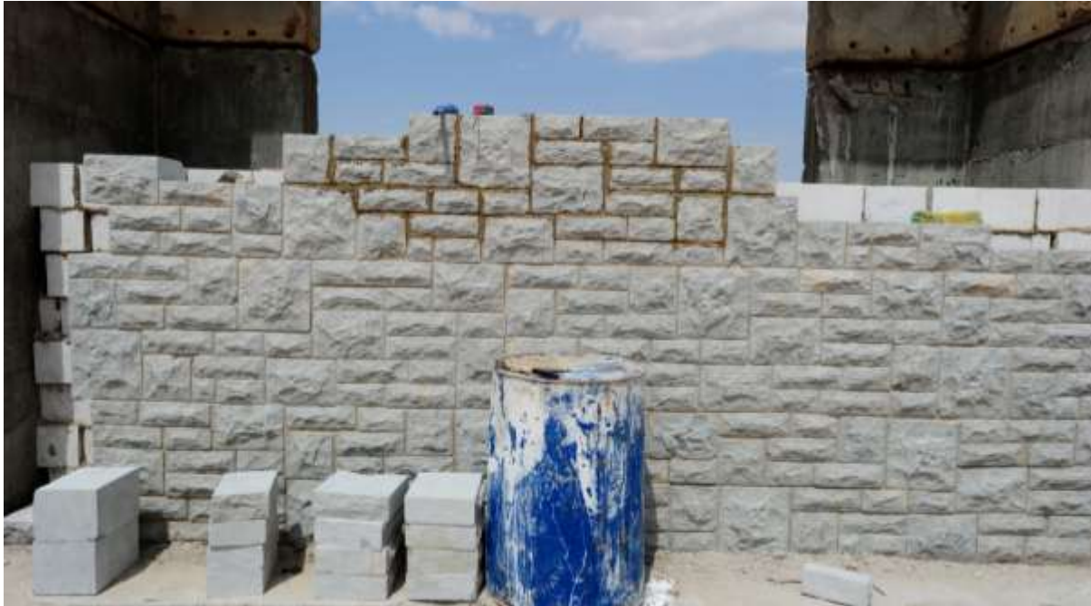
Figure 20 Historic masonry wall under construction
