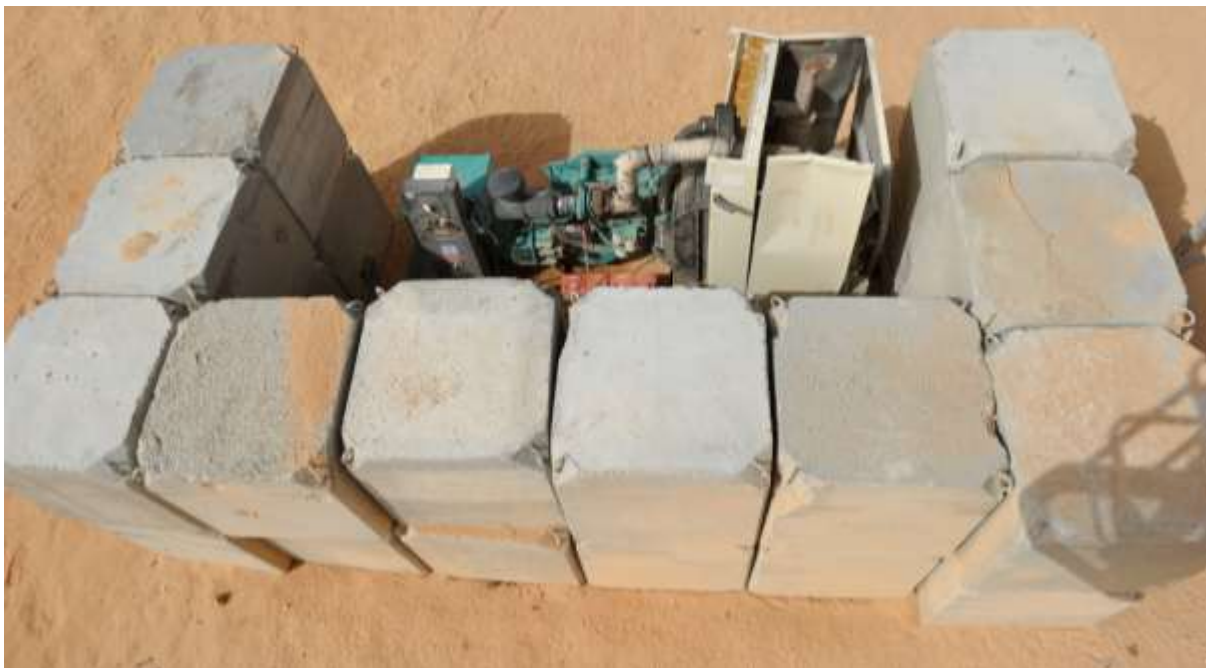
Figure 49 Generator after test
