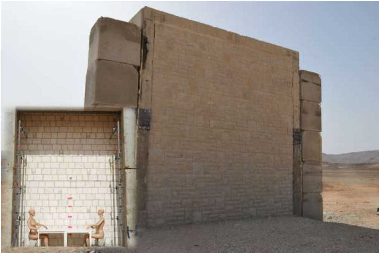
Figure 30 Historic masonry wall before test
