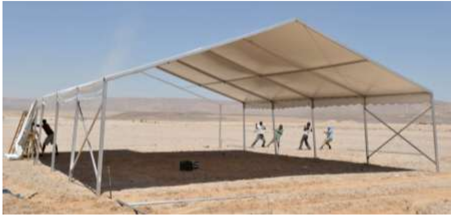
Figure 13 Tent being erected on-site
