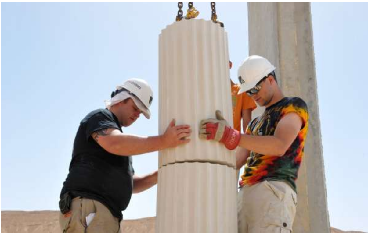
Figure 21 Neoclassical multi-drum columns under construction
